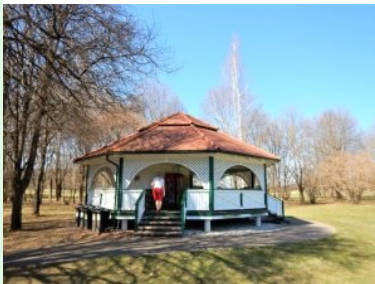
Halfway Station in Form eines Teehauses
