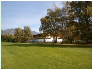
Greenkeeper House neben Fairway 12
