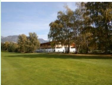
Greenkeeper House neben Fairway 12
